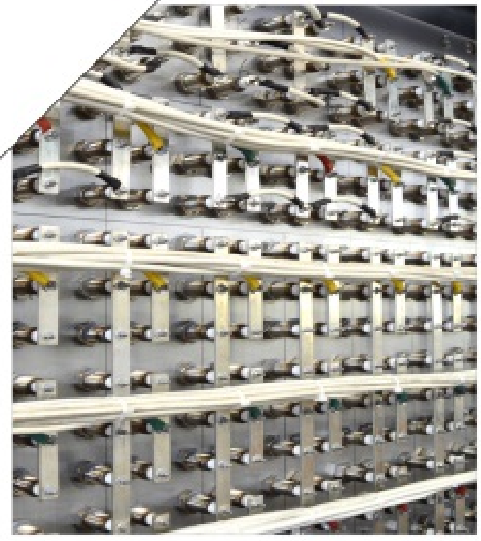
Copper bars and heat-resistant wires
